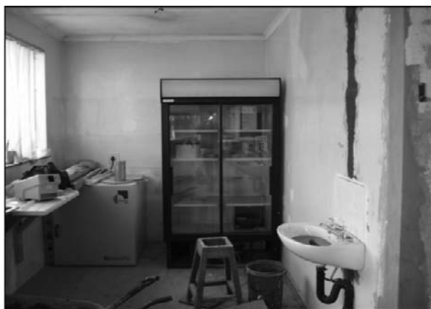
Figure 1 Tuberculosis reference laboratory, pre renovation.
